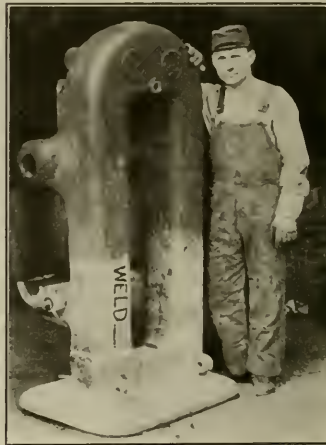
VIEW OF HEAVY STEEL CASTING AFTER WELDING.
